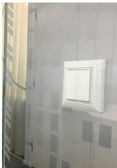
Wireless Control Panel mounted on a glass wall
