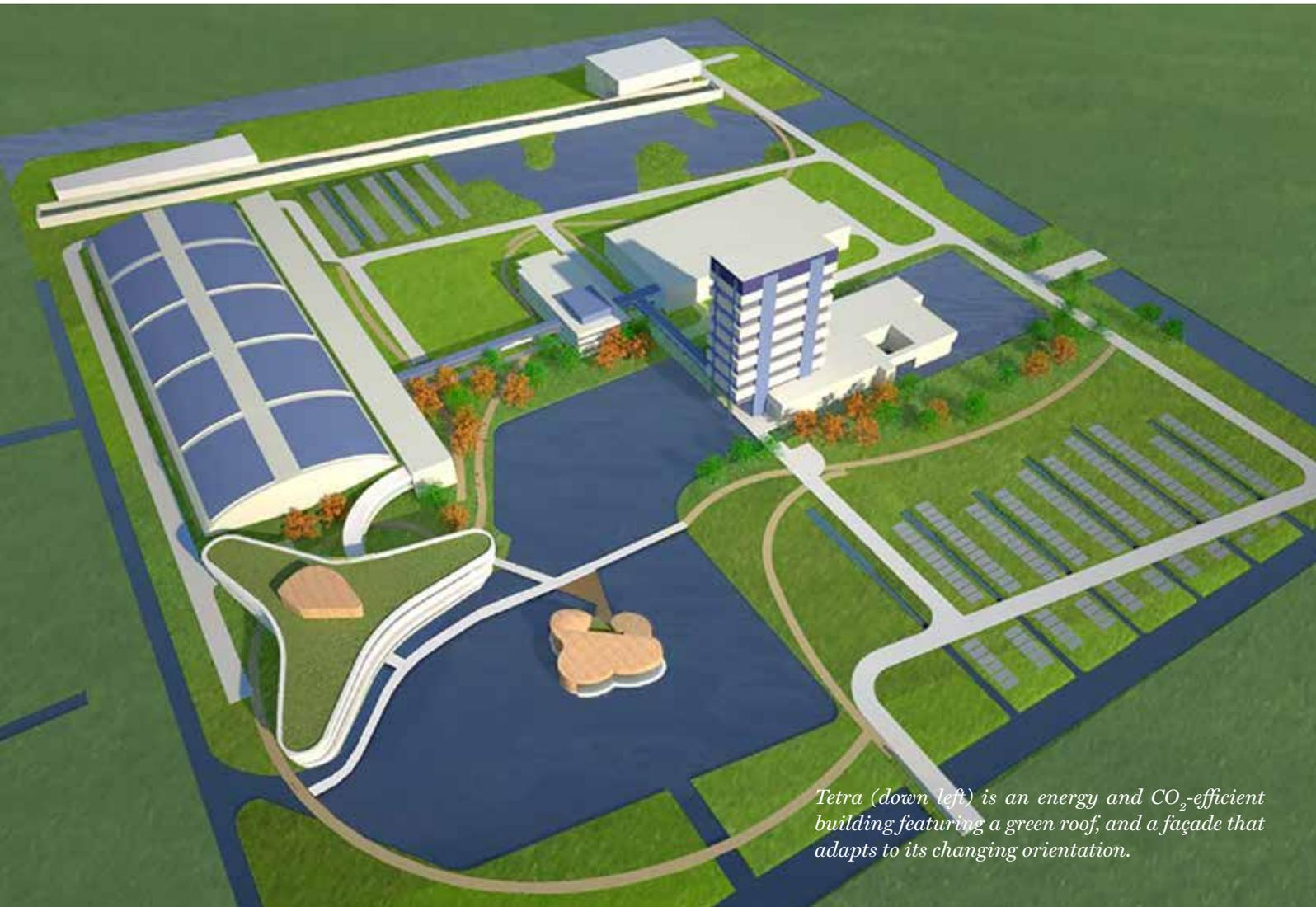
*Tetra (down left) is an energy and CO<sub>2</sub>-efficient building featuring a green roof, and a façade that adapts to its changing orientation.*
